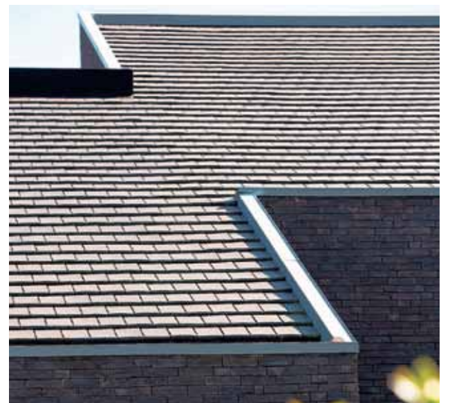
Dak met Koramic Migeon Vauban antraciet mat. Architect: Buedts & De Pape, Ertvelde
