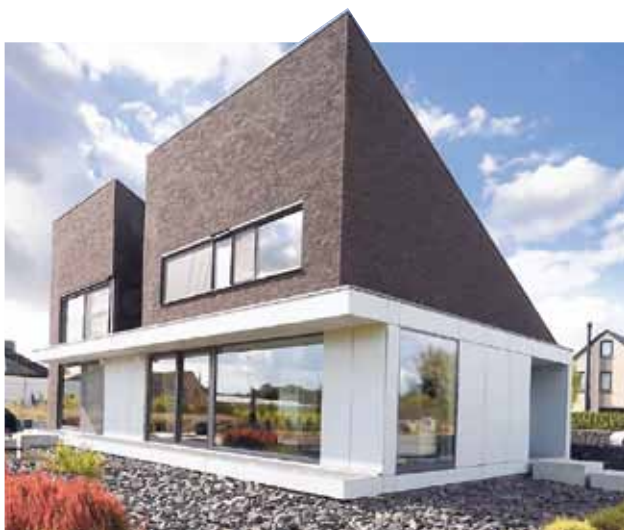
Architect: Buedts & De Pape, Ertvelde
